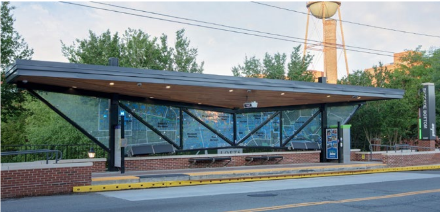
Figure 1: ADA compliant BRT station
