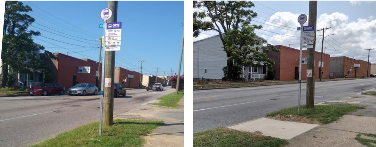
Figure 14: Before and After photos of a stop brought into ADA compliance by supplementing existing sidewalk
